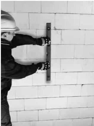
Image 18 Use a level to set out the path of the AMAXPRO soil and waste stack.
