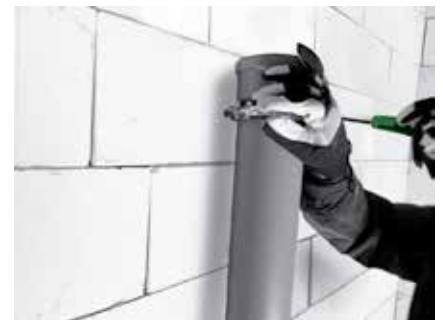
Image 23 In the last installation step, place the pipe/fitting in each bracket and bind both halves of the bracket to secure.
