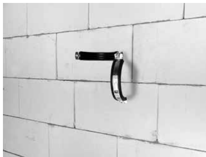
Image 22 An open pipe bracket shown ready to secure the piping.
