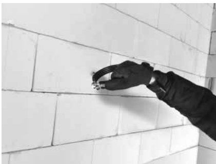
Image 21 Drive the wall plugs into the holes and install each pipe bracket by screwing it into the wall plug.
